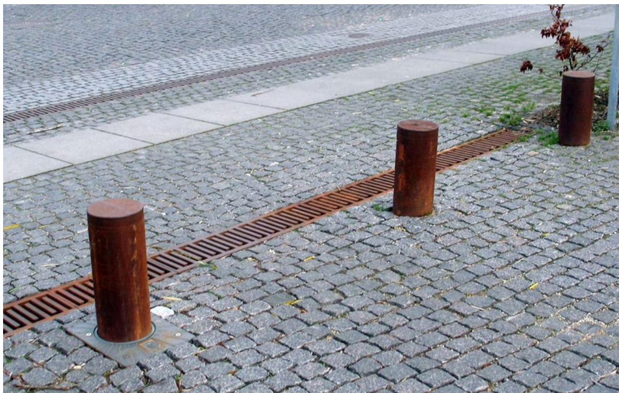
Figur 33: Heve/senke-pullerter i corten-stål. Foto: CAME Norge AS
